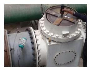
Line pressure measured using Pressure Transducer
