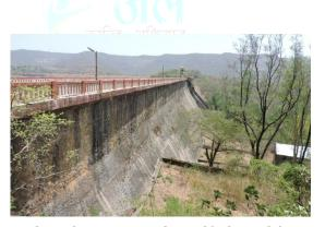
View of seepage marks at d/s face of dam
