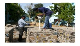
Flow time measurement and grouting of sample masonry blocks
